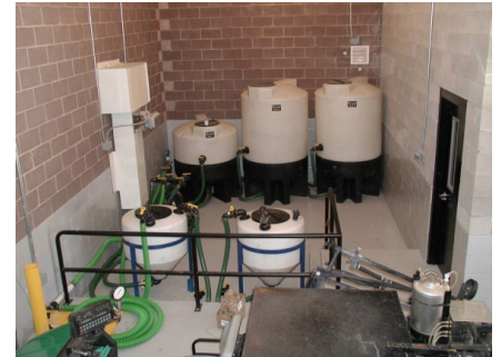
Chemical pre-mix area, utilized to pre-mix chemicals and fertilizers for spray applications.
